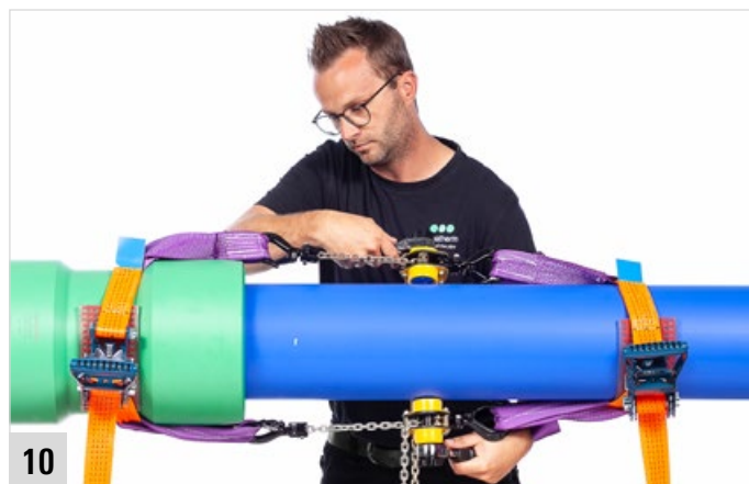
10 Pull the push-fit fitting onto the pipe end up to the marked insertion depth.
